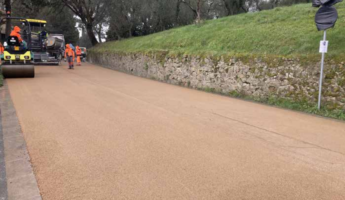
Posa in opera.
